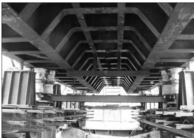
Figure 3 – Test stand (bottom view)
